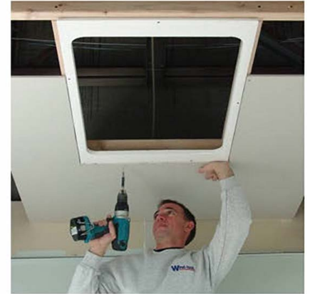
3. Hang drywall around the panel frame.
