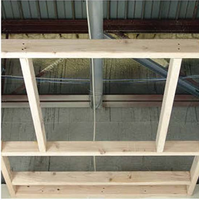
1. Frame out location of the panel.
