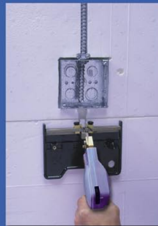
Cut the wire channel with bendable blade material
