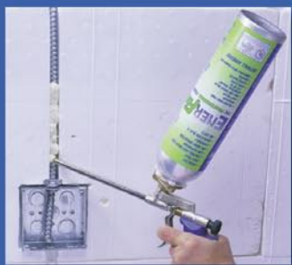
Fill in channel with EnerFoam
