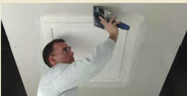
4. Tape and apply drywall compound.
