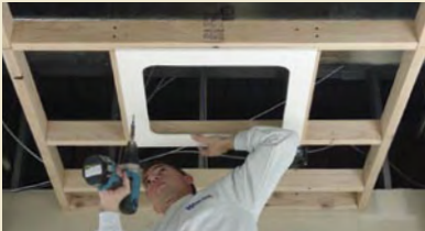
2. Mount Stealth surround with drywall screws.
